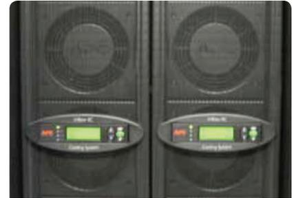
*By placing the cooling directly where it is needed (washing the face of the servers), and recirculating the discharge heat before it mixes with the remaining space, the Markley Group gets optimal efficiencies.*
