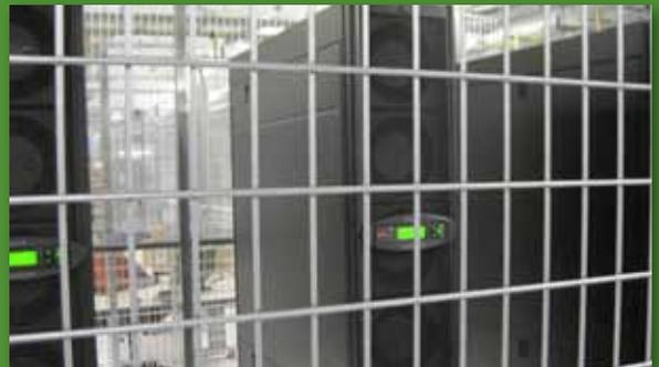
By placing the cooling directly where it is needed, (washing the face of the servers) and recirculating the discharge heat before it mixes with the remaining space, the Markley Group gets optimal efficiencies.
